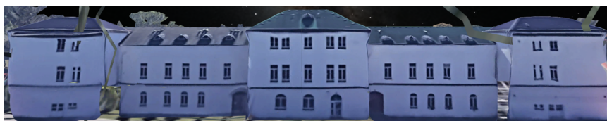
Figure 5.9: Front-side view picture of the back side of Palata. Picture taken from the Google Earth.
